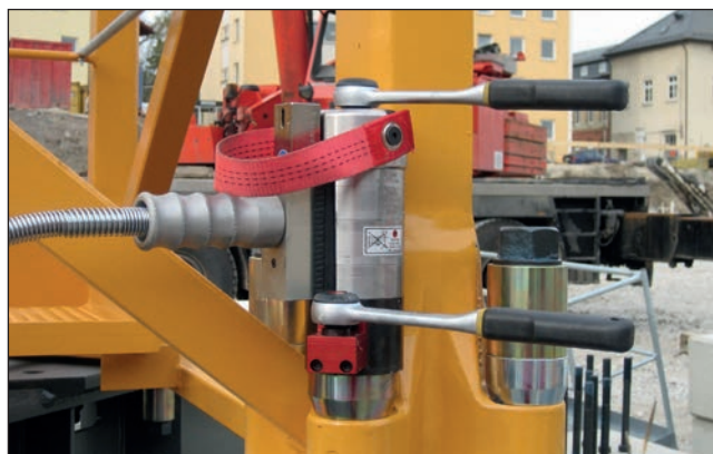
Tower segment bolt connection at tower crane.
