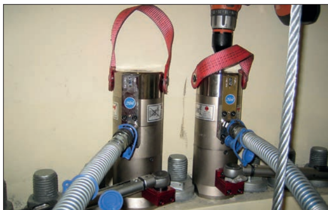
Tower segment bolt connection at wind turbine.
