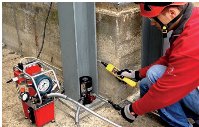
Foundation bolt connection.
