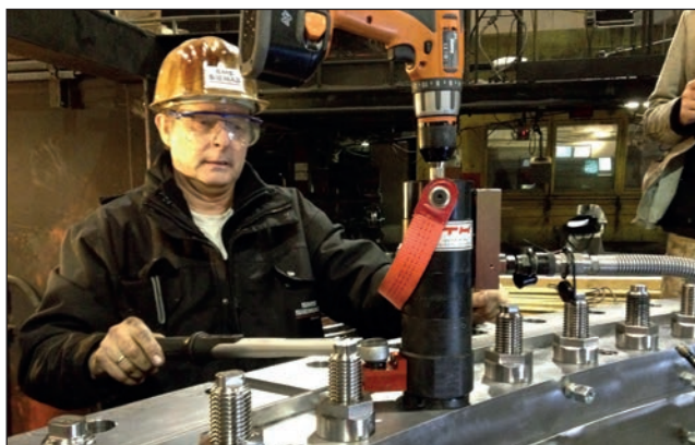
Ladle turret bolt connection.
