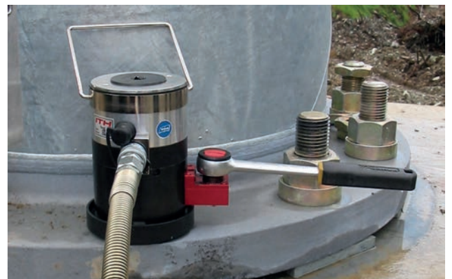
Foundation bolt connection.
