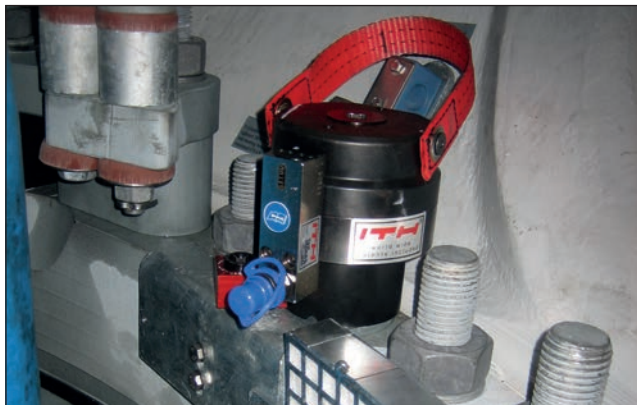
Tower bolt connection.
