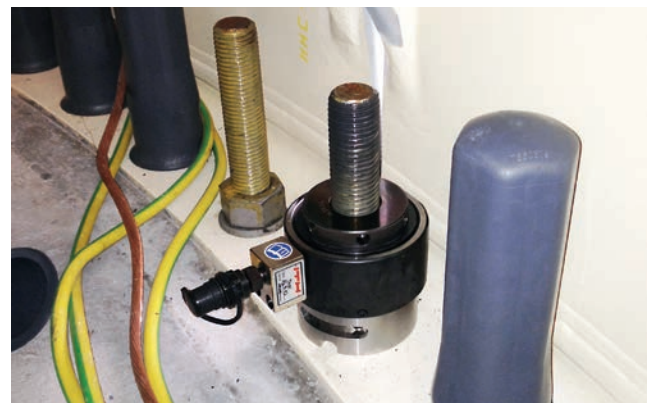
Foundation bolt tensioning.
