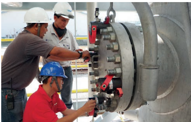
Assembling of BTC type ES on an ANSI flange.
